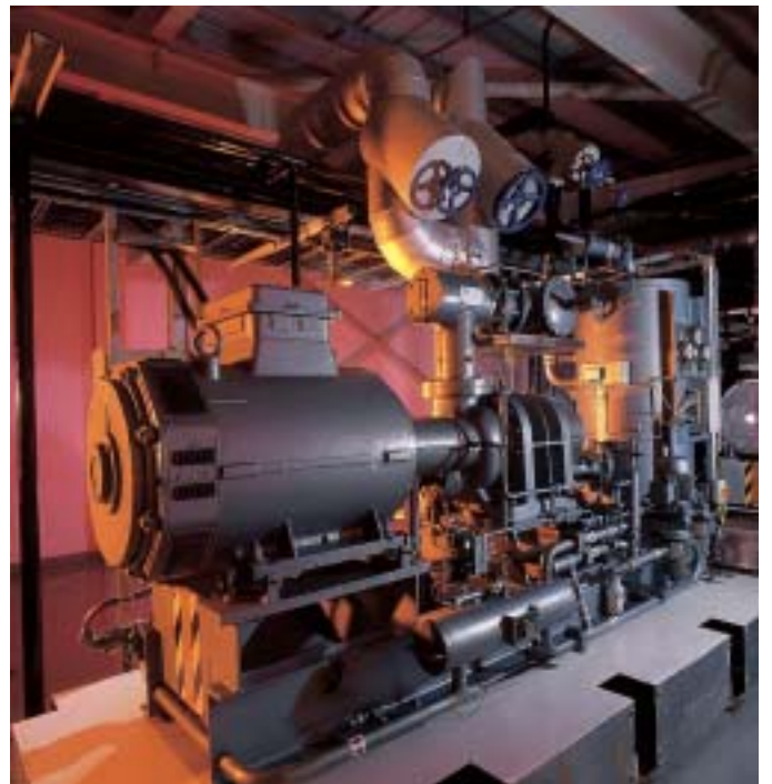
Refrigeration system installed at a dairy plant in the United Kingdom. Screw compressors, made by Grasso, are the heart of this installation. Revalco contributed the valves.
